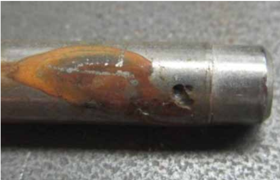
Figure 9: Pitting with related staining on a 410 stainless steel Solid Pin.
